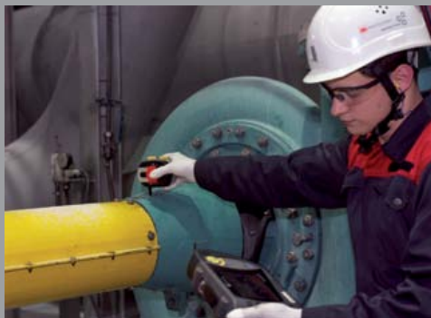
Vibration measurement The good alignment should be confirmed by reduced vibration values.
