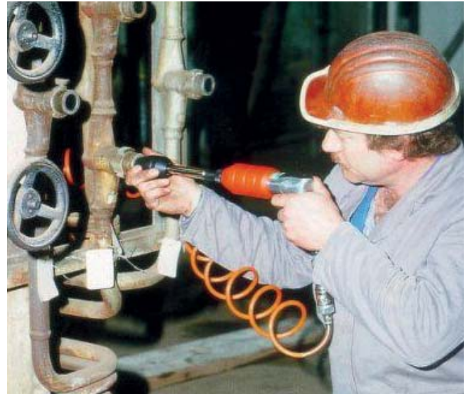
KVS grinding on-site
